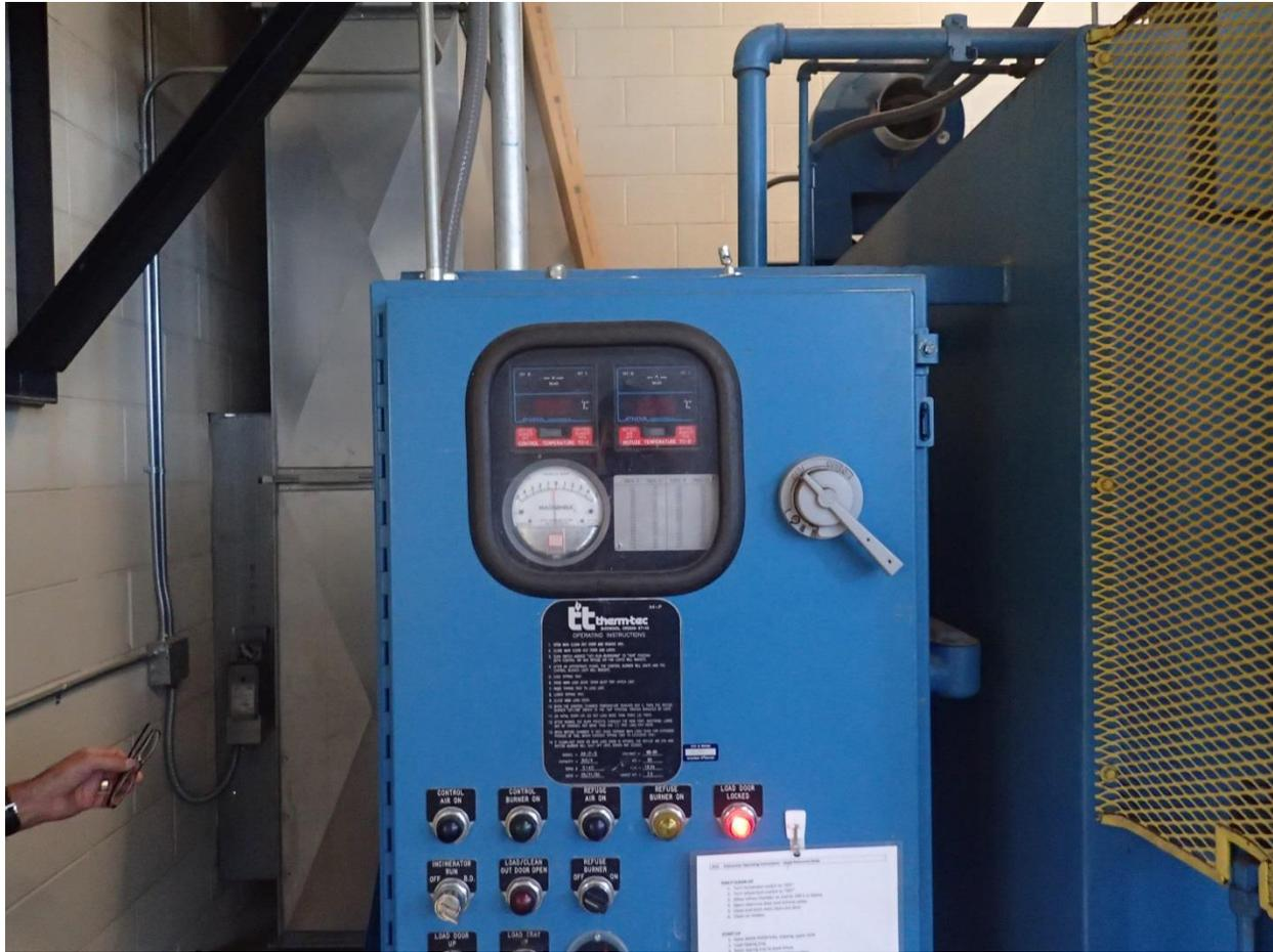
Figure 2. Incinerator Control Panel and Temperature Monitor
